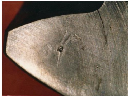
Figure 43 - Bending fatigue crack
